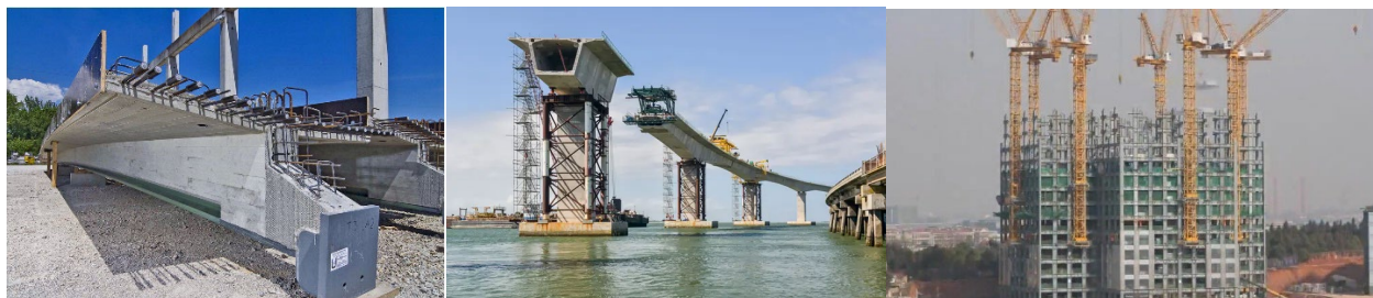
Figure 21 – (in order of left to right) – Prefabricated Road, Prefabricated Bridge, Prefabricated Skyscraper. The start to finish construction time of the 57-story skyscraper at the right was 19 days. 104
